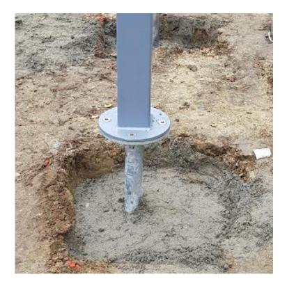
6 - Tighten the security bolts completely ONLY when the posts are level, **use Loctite:**
