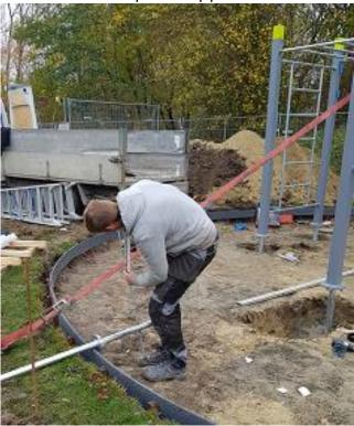
5 - Add fast-setting concrete into the hole. It depends on the condition of the soil and the size of the hole how much this should be. For most types of soil the dimensions of the hole should be 500x500x750mm; this gives around 0.12 m3 of concrete. When the soil is very loose (like sand) a bigger hole and more concrete is advised.
