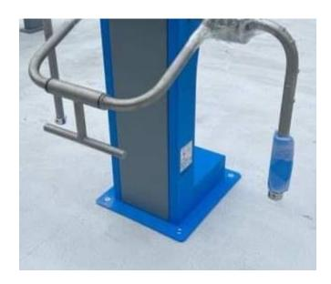
BEFORE APPLYING WET POUR OR ARTIFICIAL GRASS MAKE SURE THAT THE COMPLETE UNIT IS LEVEL, STABLE AND CORRECTLY INSTALLED!
