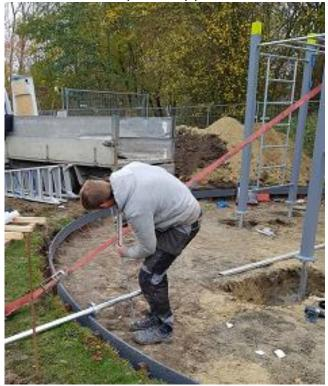
5 - Add fast-setting concrete into the hole. It depends on the condition of the soil and the size of the hole how much this should be. For most types of soil the dimensions of the hole should be 500x500x750mm; this gives around 0.12 m3 of concrete. When the soil is very loose (like sand) a bigger hole and more concrete is advised.
